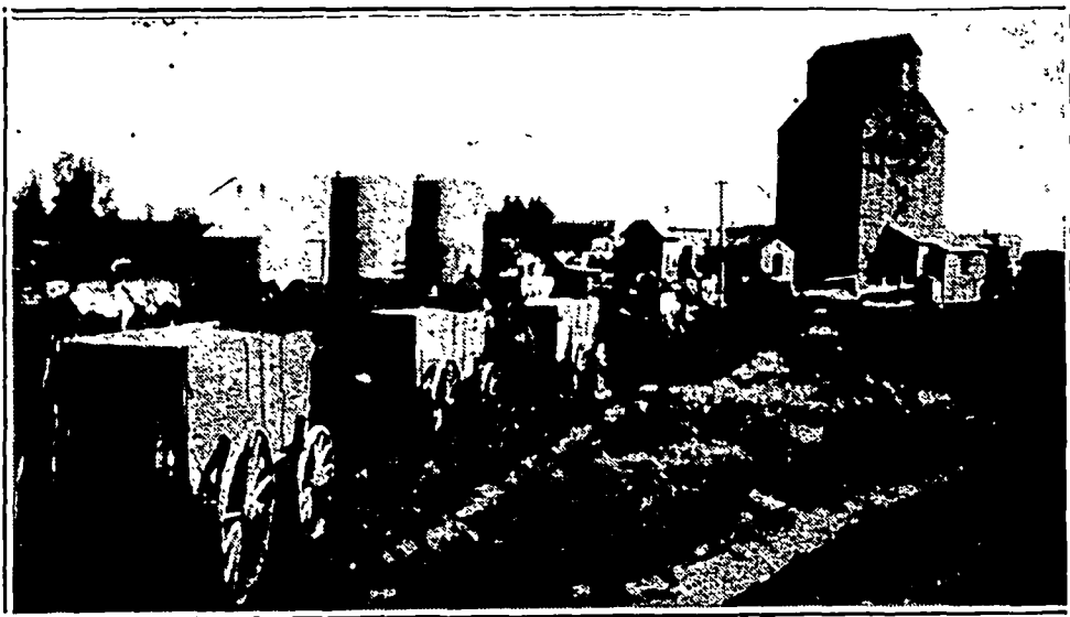
A-Line-Up at Waskada Pool Elevator
